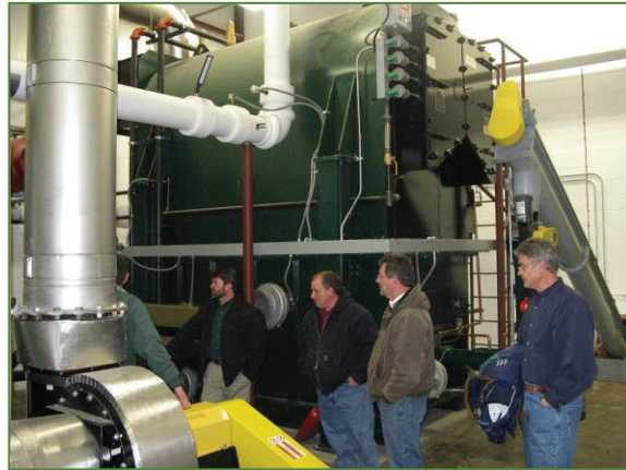
Commercial scale wood boilers are large systems that supply hot water or steam to the building or facility they serve.
